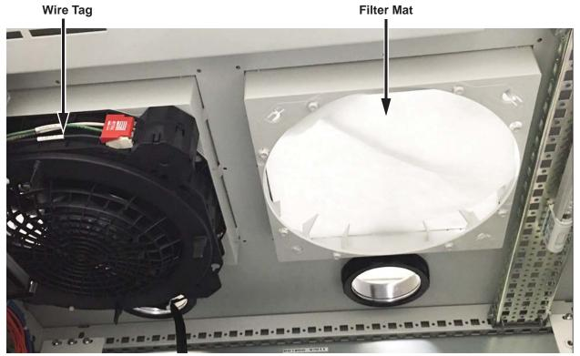
Figure 7: Fan removed with filter mat exposed.
